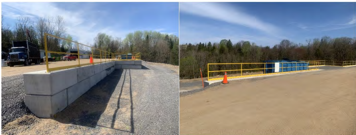
Plate 8: Asset ID SW6 – Waste Site Transfer Station Retaining Wall
