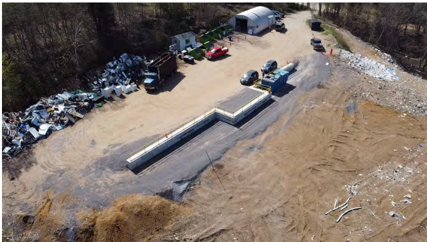
Plate 1: Overhead View of Wollaston Waste Disposal Site Transfer Station and Approved Waste Disposal Area (AWDA)
