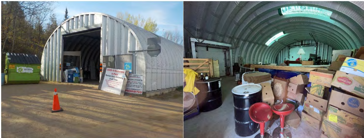
Plate 7: Asset ID SW5 – Waste Site Recycling Building
