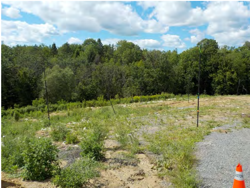
Plate 3: Photograph of New Grade Stakes Installed on July 26, 2022
